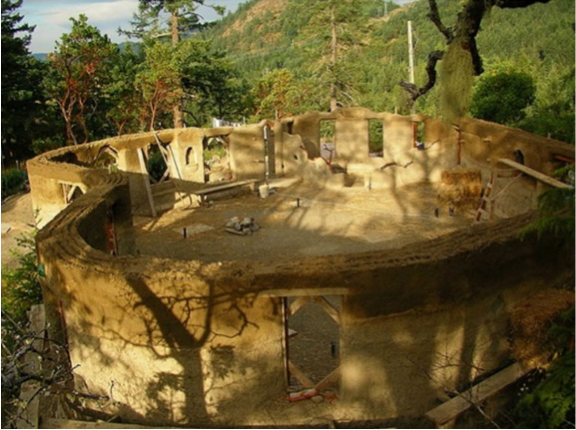
Figure 5: Eco-Sense Walls at Six Weeks
