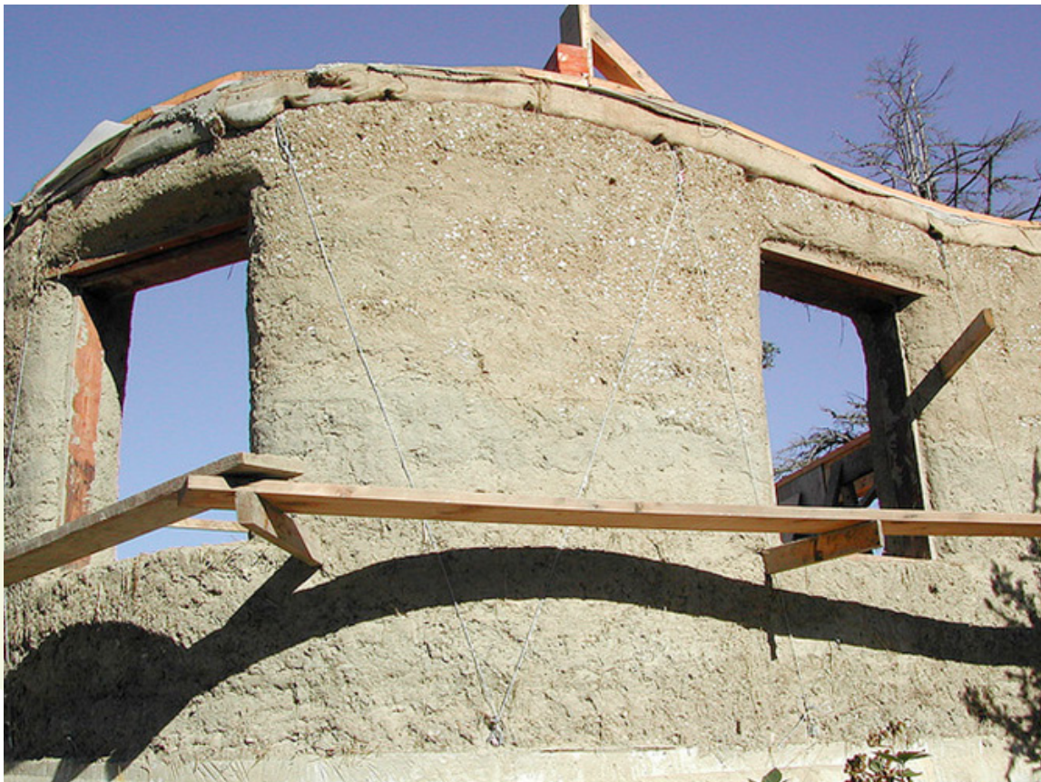
Figure 21: Mass Wall with Tension Cables
