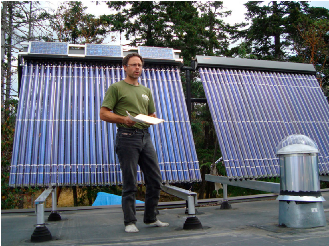
Figure 11: Eco-Sense Solar Hot Water Class
