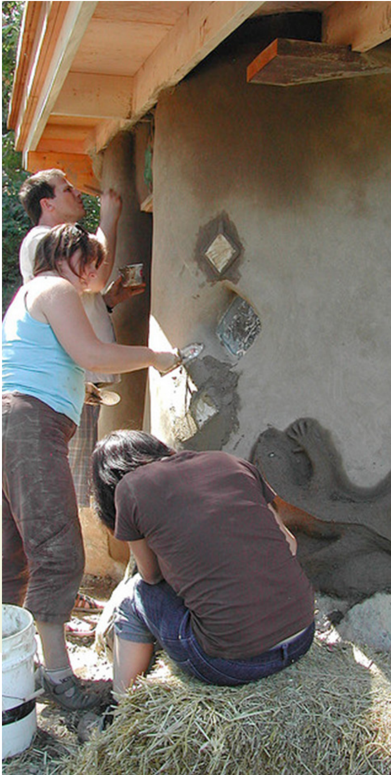
Figure 7: Cob Cold Storage
