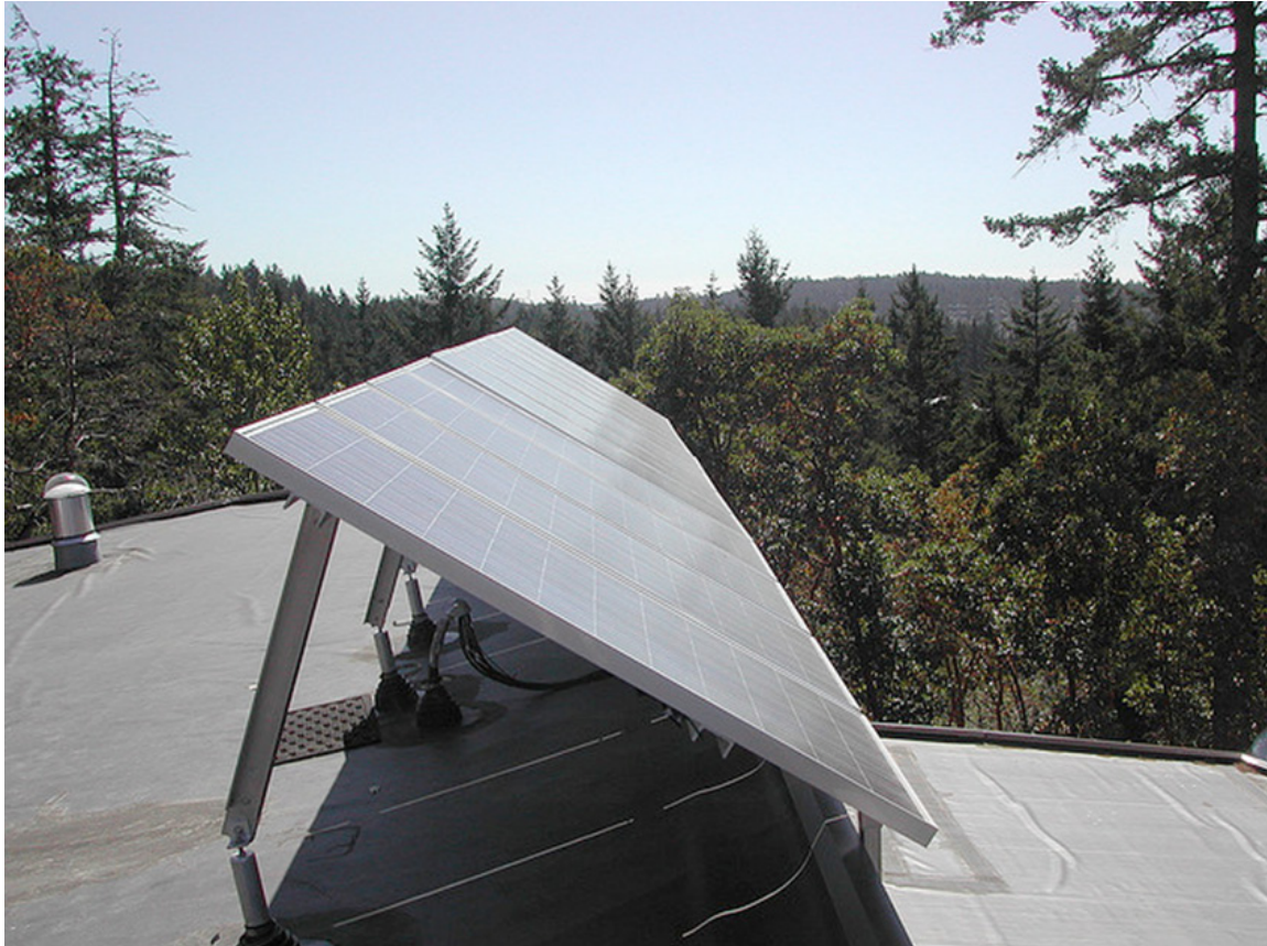
Figure 14: Photovoltaic system before Living Roof was planted
