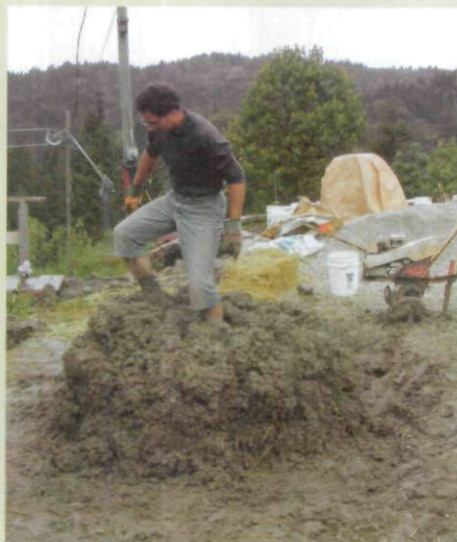
Emily, then age 5 (left), holds up a glob of cob, ready to slap into place as the house goes under construction. Meanwhile, Gord demonstrates the similarities between crushing grapes and the traditional way of mixing cob (above); he soon streamlined the method with the help of a roto-tiller (below).
