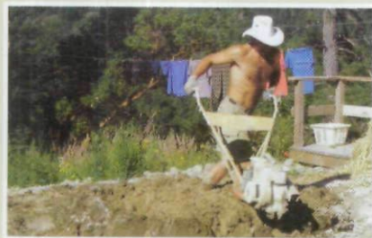
Emily, then age 5 (left), holds up a glob of cob, ready to slap into place as the house goes under construction. Meanwhile, Gord demonstrates the similarities between crushing grapes and the traditional way of mixing cob (above); he soon streamlined the method with the help of a roto-tiller (below).
