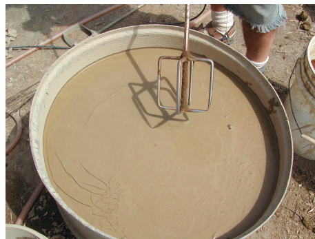
Clay slip soaking in half barrel. Different clays can take different amounts of time to fully hydrate
