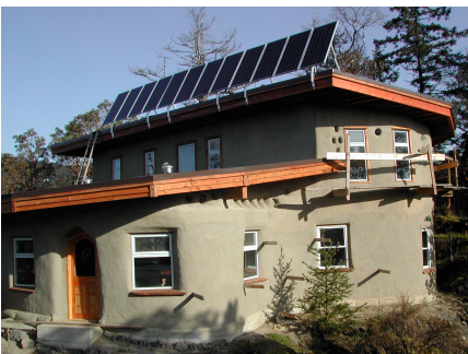
Brown coat on cob. We could have quit here but added finish lime plaster coat.
