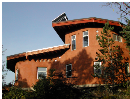
Earth plasters on Cob building One coat Clay plaster One coat Lime plaster
