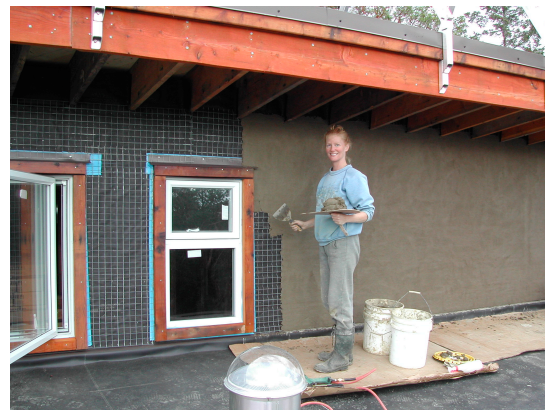
Brown coat on wood frame construction. Prepped with tar paper and stucco wire. Two coats of lime plaster went on top.
