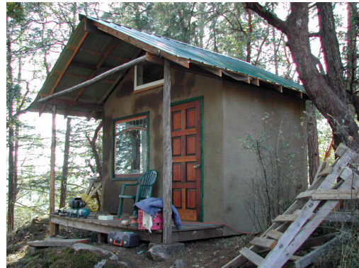
Earthen plaster on wood frame building. Two coats of clay plaster
